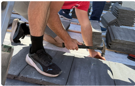
Post-storm repair, Mesa. Microburst lifted multiple tiles in a single course.
